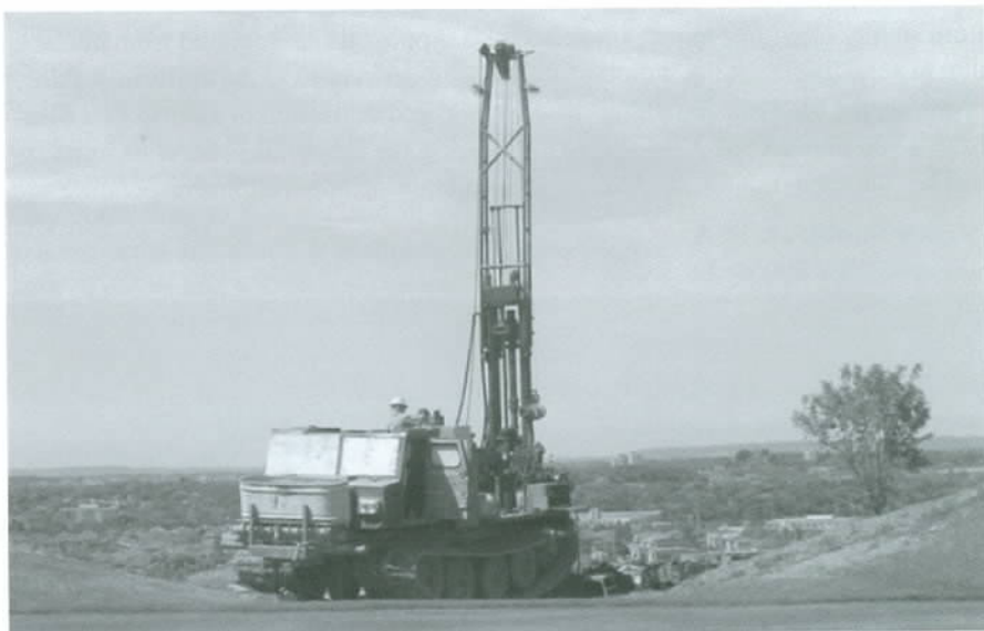
Installation of a gas well on the BraeBen Golf Course.
